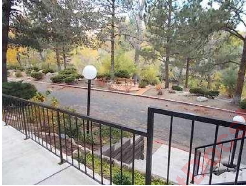
Painting of all Wrought Iron is done by the Maintenance Supervisor every 5 years or when needed. Future Replacement of the Pole Light Fixtures has been included in the Study.
