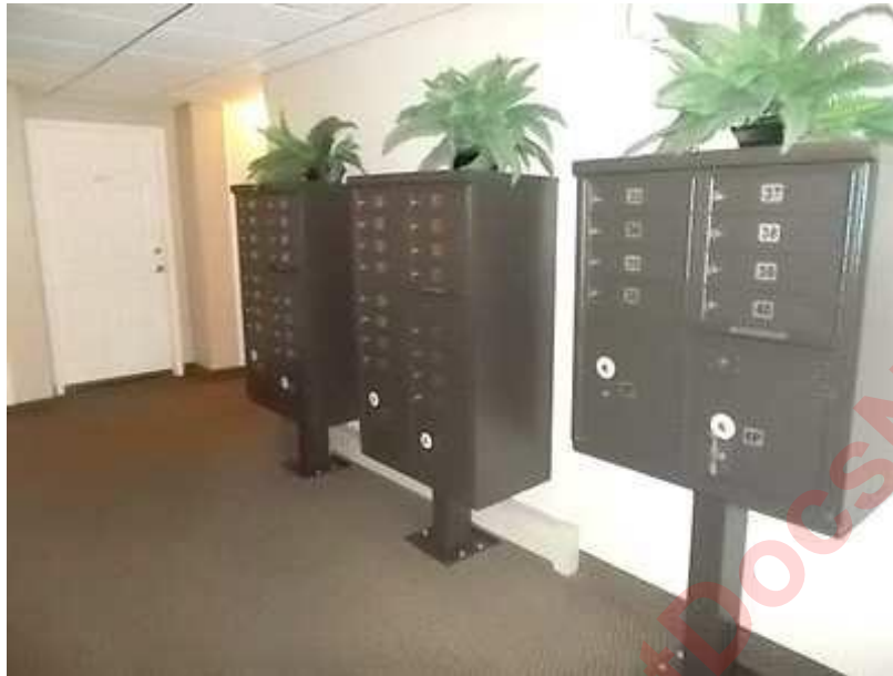
The Mail Boxes are Maintained by the Homeowners Association. The Estimated Useful Life when New is approximately 20 years. Replacement has been included in this Study.
